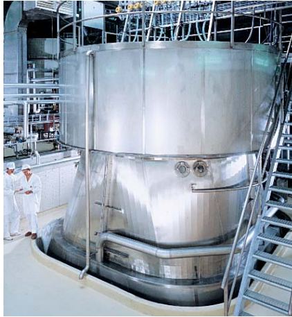
Top of drying chamber showing air disperser
