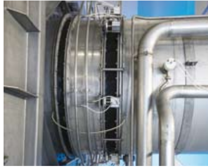
Vapour tight damper isolates and keeps SANICIP™ dry during wet cleaning of other parts
