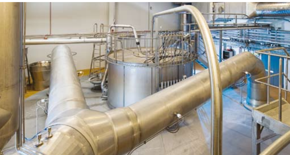
Air exhaust ducting from top of spray drying chamber equipped with CIP nozzle
