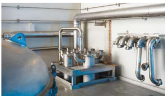
Vertical holding tubes make CIP and inspection easy
