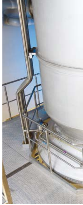
An evaporator calandria with 16-18m tubes. Coverage of each tube is improved and fouling/deposits are reduced. CIP is fast and effective
