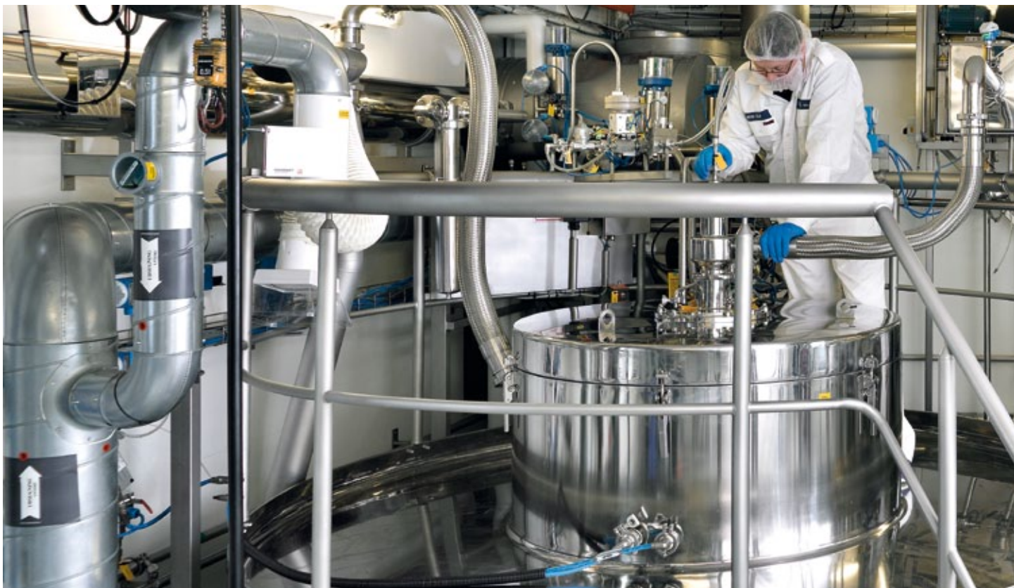
PSD-4 Chamber roof with gas disperser and top of bag filter.
