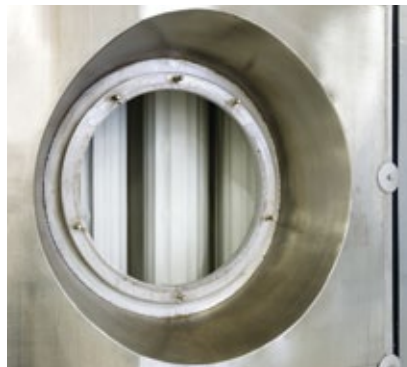
Filter bags after wet cleaning
