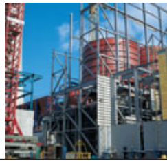
Left: Erection of an SDA plant in Denmark.
