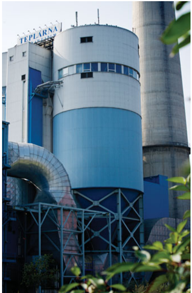
Large SDA module at a lignite coal fired power plant in the Czech Rep.
