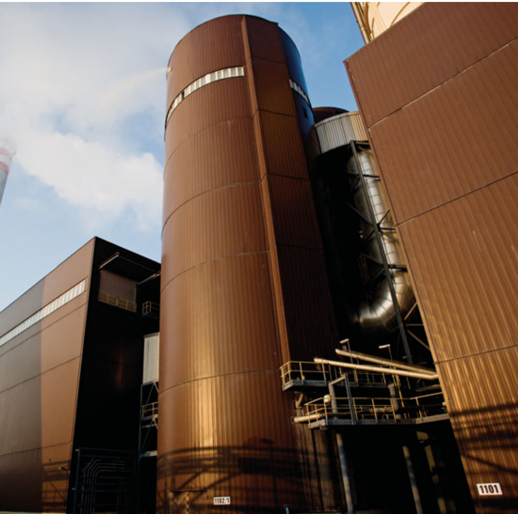
Two parallel absorber modules treat the flue gas from 8 lignite fired boilers installed in the Czech Rep.
