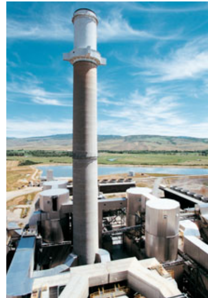
Adjacent SDA's at two parallel coal fired units in the USA.
