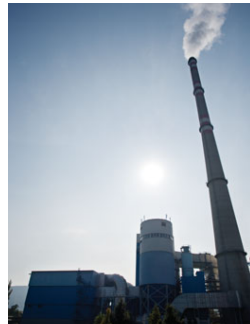
530 MW e lignite fired power plant in the Czech Rep.
