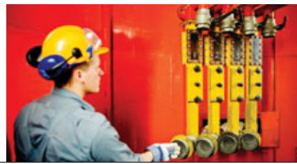
An activated carbon injection system installed at a Danish waste facility with 4 incineration lines.
