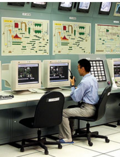
Operation of an SDA plant is typically handled from the central control room, without extra staffing.
