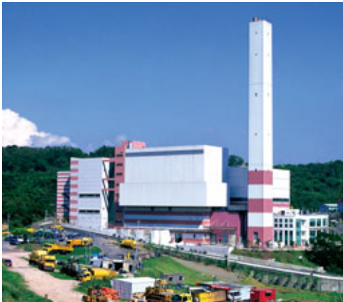
A Taiwanese waste incineration facility with two GEA Niro SDA systems, 2 x 300 TPD.
