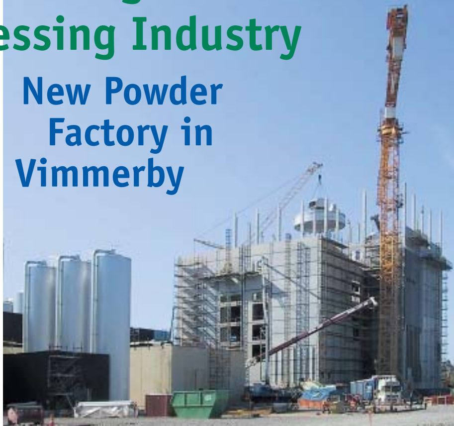
Part of drying chamber being lifted into the building.
